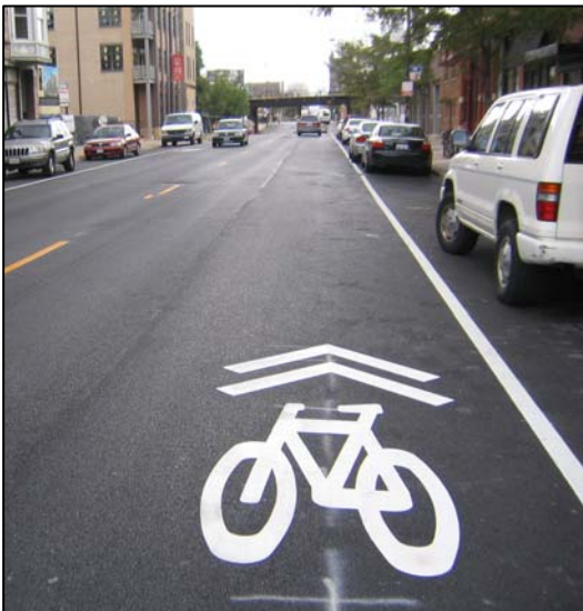
A new shared lane marking (below) on Milwaukee Avenue alerts motorists and cyclists to the road's shared status.
